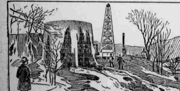
UNABLE TO CONTROL THE FLOW OF OIL.
