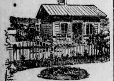
HOUSE WHERE HOT WATER IS FURNISHED TRAVELERS ON SIBERIAN RAILWAY.
