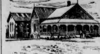
CHURCH AND PARSONAGE TYPICAL OF THE TRANSVAAL.
