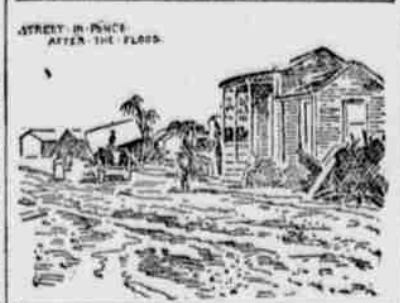
STREET IN PONCE AFTER THE FLOOD.
