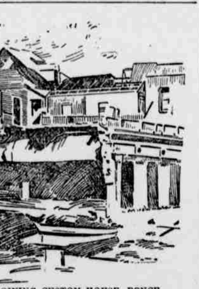
WRECKED CAFE IN PLAZA ADJOINING CUSTOM HOUSE, PONCE.
