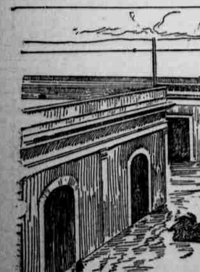
STREET IN ARECIBO, PORTO RICO, DURING THE HURRICANE, SHOWING HEIGHT OF WATER ON THE HOUSES.
