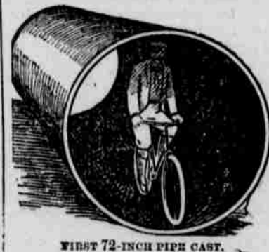
FIRST 72-INCH PIPE CAST.
