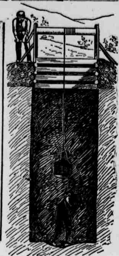
2. DIGGING AND DUMPING.
