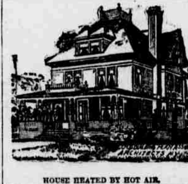
HOUSE HEATED BY HOT AIR.
