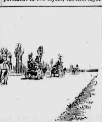
A MECKLENBURG COUNTY (NORTH CAROLINA) ROAD.
