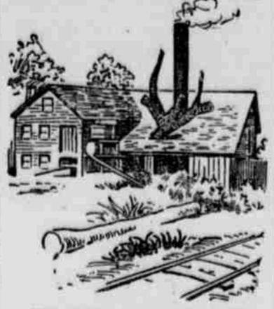
MILL WITH A TREE IN ITS ROOF.
