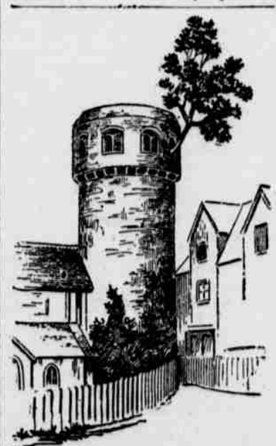
TREE ON NORWICH TOWER.
