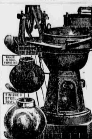
JUMBO, the Alexander Improved Cream Separator; capacity 2500 to 4000 pounds per hour; two horse power will run it. Also new model HAND SEPARATOR for the sale of which AGENTS are WANTED in every section. Manufacturers of complete line of machinery and supplies for butter and cheese factories. Send for catalogue, DANIS & RANKIN BUILDING AND MFG. CO., 310 to 324 West Lake Street, Chicago, Illinois.
