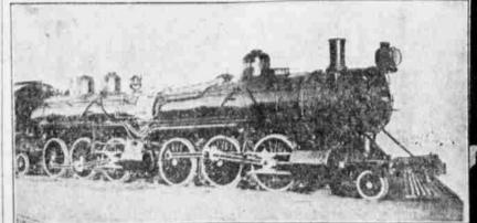
This locomotive has been built by an American railroad company and tested but a few days ago. Its pecularity consists in the boffer which on account of its length had to be jointed in the middle, to enable it to take all the curves of the road. Conservatively estimated this locomotive with the tender together is about 75 feet long. This is the first and so far the only notive of this kind.
