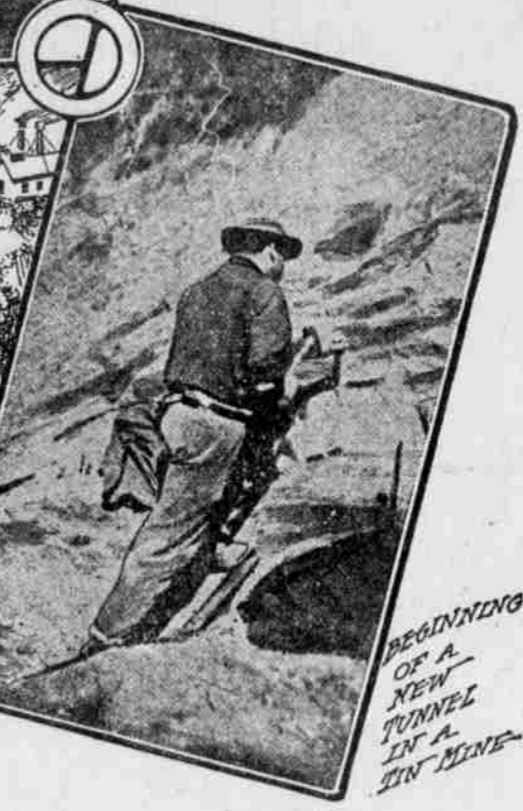
BEGINNING OF A NEW TUNNEL IN A TIN MINE
