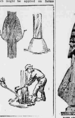
Reinforcing Poles with Concrete. where posts in a barn are rather difficult to displace and are rotting away near the surface of the ground.
