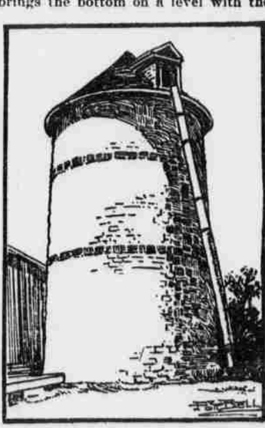
A CEMENT BLOCK SILO.
