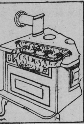
Odor Goes Up the Chimney.
