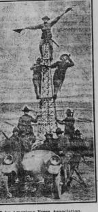
The newest armored auto also has a steel tower, which can be raised on the principle of a fire ladder and on the principle of a first latter and employed for signaling, observation, outpost station work and in military field wireless. The United States may soon be equipped with this "tank," which has been tested by the New York national guard.
