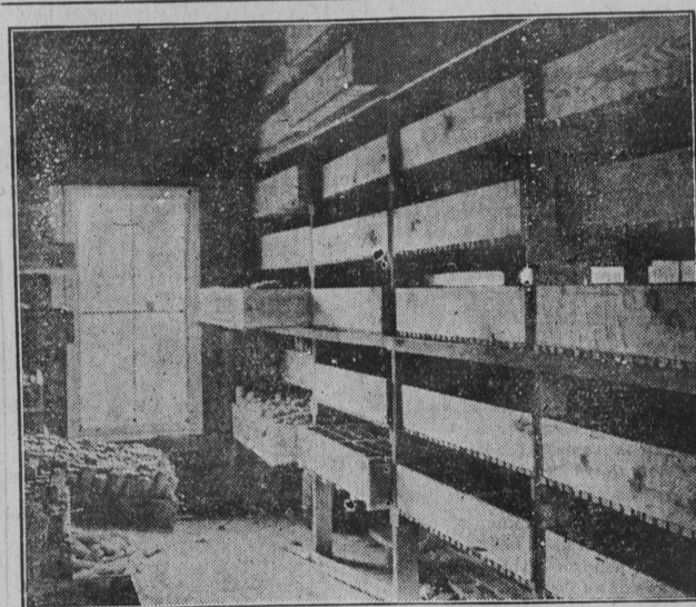
Interior View of Seed Corn House at Piketon, Ohio.
