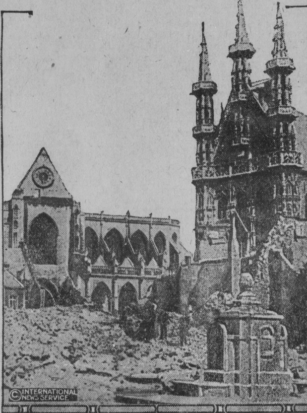
The magnificent cathedral of Louvain, the interior of which was utterly wrecked by the German troops, although the outer walls remain standing. At the right is the beautiful old hotel de ville, or town hall, which almost alone of the city's buildings was spared.
