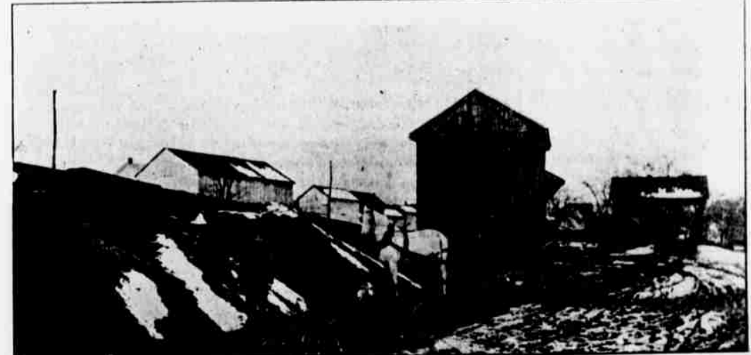
VIEW OF STEININGER BROTHERS COAL YARD.
