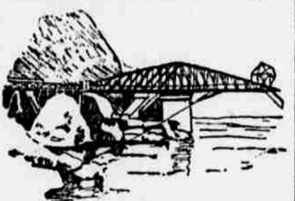
CANTILEVER WHARF. (Recently Completed at Salta-Cabelle, Spain.)
