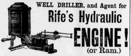
to It is a new and marvelous invention. Just the thing you want for elevating a continuous supply of water frrom springs or branches. It is self-operating, simple in construction and unsurpassed in durability. They are now being placed in every State in the Union and are wanted in every county, town and village. We challenge the world to produce its equal. Must prove satisfactory before payment is made. For further information write for illustrated catalogue.
