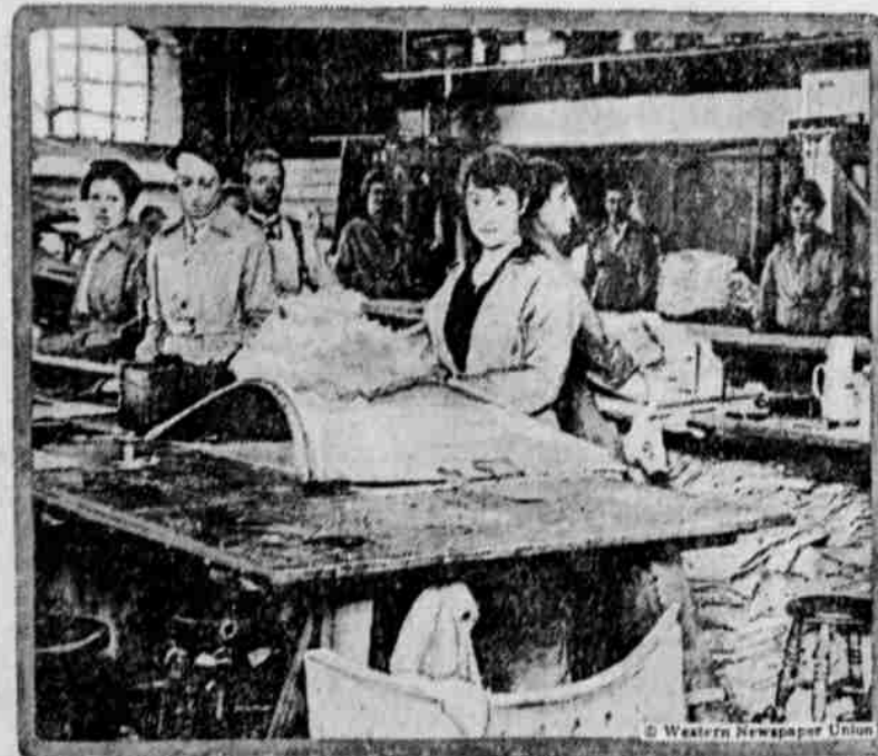
Upholstering department of a great airplane factory in England where girls are putting on the fabric covering for the decks and fuselage.
