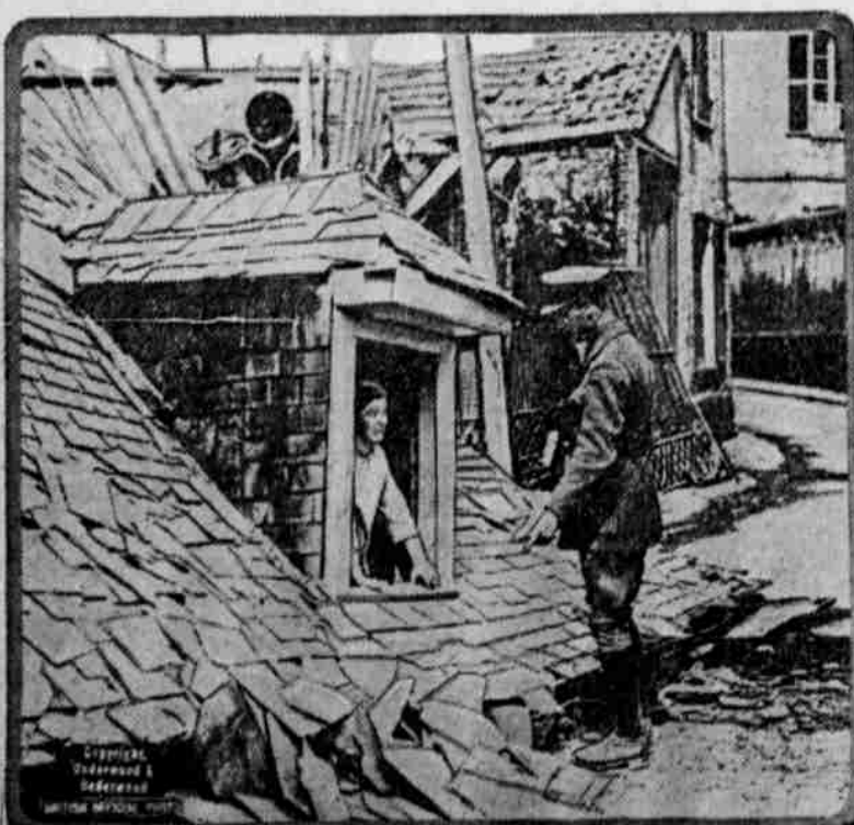
In answer to the British Tommie's remark, "I see you've moved," this young lady replies: "Yes, so I have, but not willingly." The cause of her remarkable predicament and that of the house was a shell from a Boche gun on the western front which exploded near the foundation, causing the walls to cave in and thereby bringing the attic down to the level of the street.
