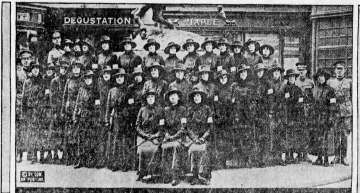
These are the first of the American telephone girls who are going to operate the switchboards for our soldiers in the fighting lines, photographed on their arrival for duty in France.
