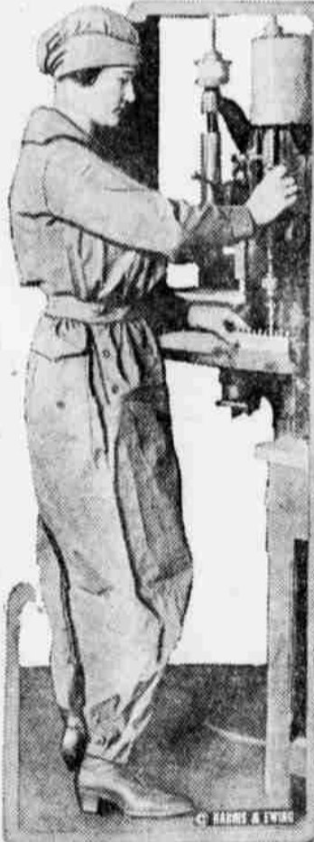
This costume of especially designed blouse, overalls and cap, has been adopted by the United States government for use of women workers in government munitions plants. A committee of women workers at the Frankford arsenal designed it. Experience has shown the advantage of its safety features.
