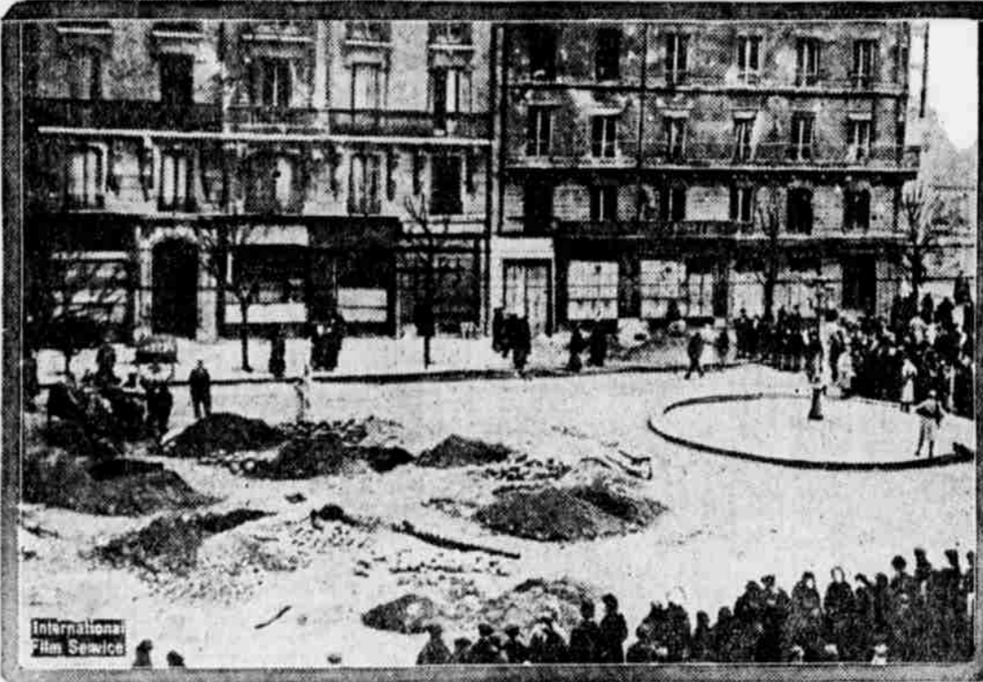
One of the streets in Paris showing the damage caused by a 200-pound torpedo dropped from a raiding Gotha on the night of January 30. Great holes many feet deep were made by the torpedoes, and the buildings in the background were badly injured.
