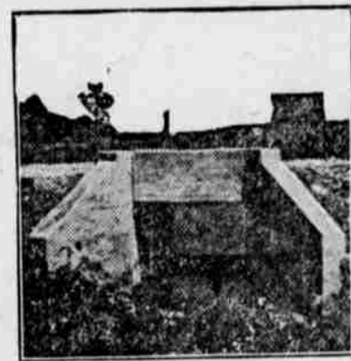
Culvert Built of Concrete.
