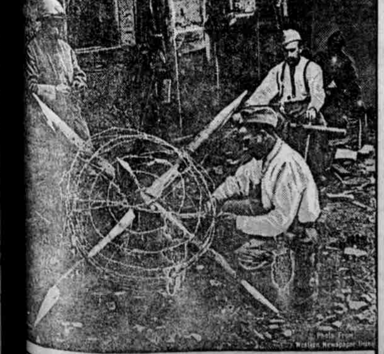
Entanglements such as these soldiers are making are used by the French with good results in places where posts cannot well be set up.
