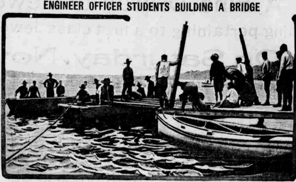
ENGINEER OFFICER STUDENTS BUILDING A BRIDGE The young engineering officers whom the government is training at the camp at Belvoir, Va., get not only theory, but actual practice in engineering problems. They are seen here constructing a light pontoon bridge.
