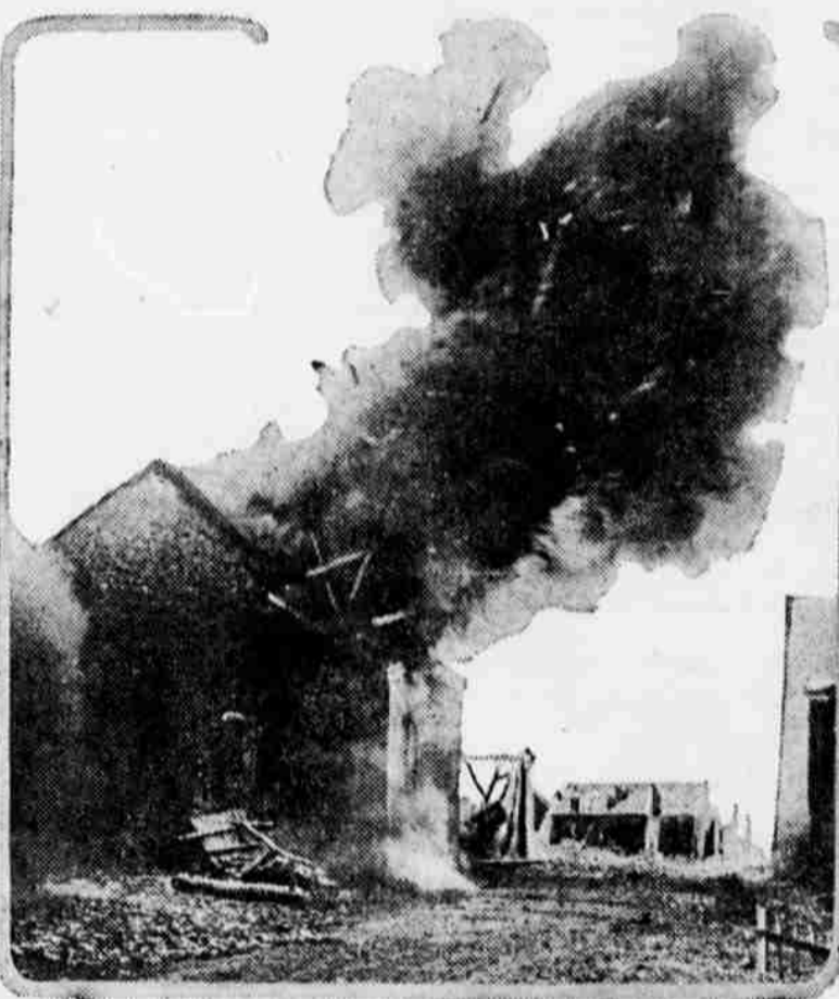
This remarkable photograph, taken recently during the British advance, shows the actual explosion of a large house in a French village, where the Germans had stored a great quantity of ammunition. Before their retreat they set fire to this and other nearby buildings and the great explosion occurred only a few seconds before the British arrived on the scene.
