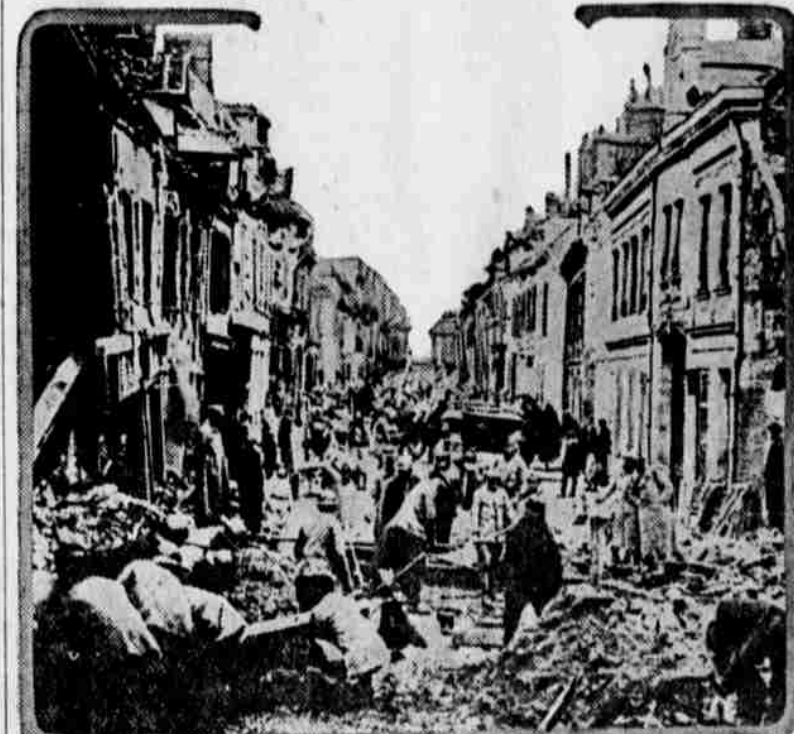
As fast as the Germans are driven back from the territory they have been holding in northern France, French engineers are rushed in to repair the devastation wrought by the Germans "for military purposes." This photograph of engineers at work in Noyon gives a vivid idea of the unnecessary havoc wreaked on the towns by the Kaiser's retreating forces.
