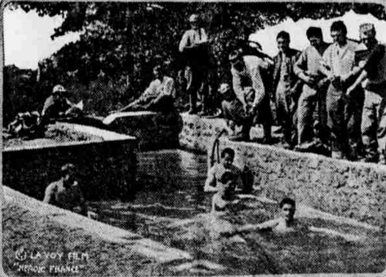
This stone swimming tank was built by the Zouaves two miles in the rear of the trenches.
