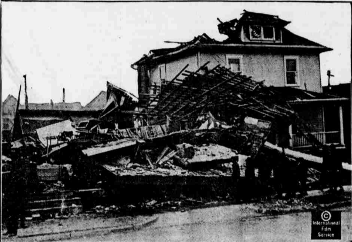
Drug store and dwelling at Eighteenth street and C avenue, Newcastle, Ind., wrecked by the terrific tornado that swept through that part of Indiana, leaving death and destruction in its wake.
