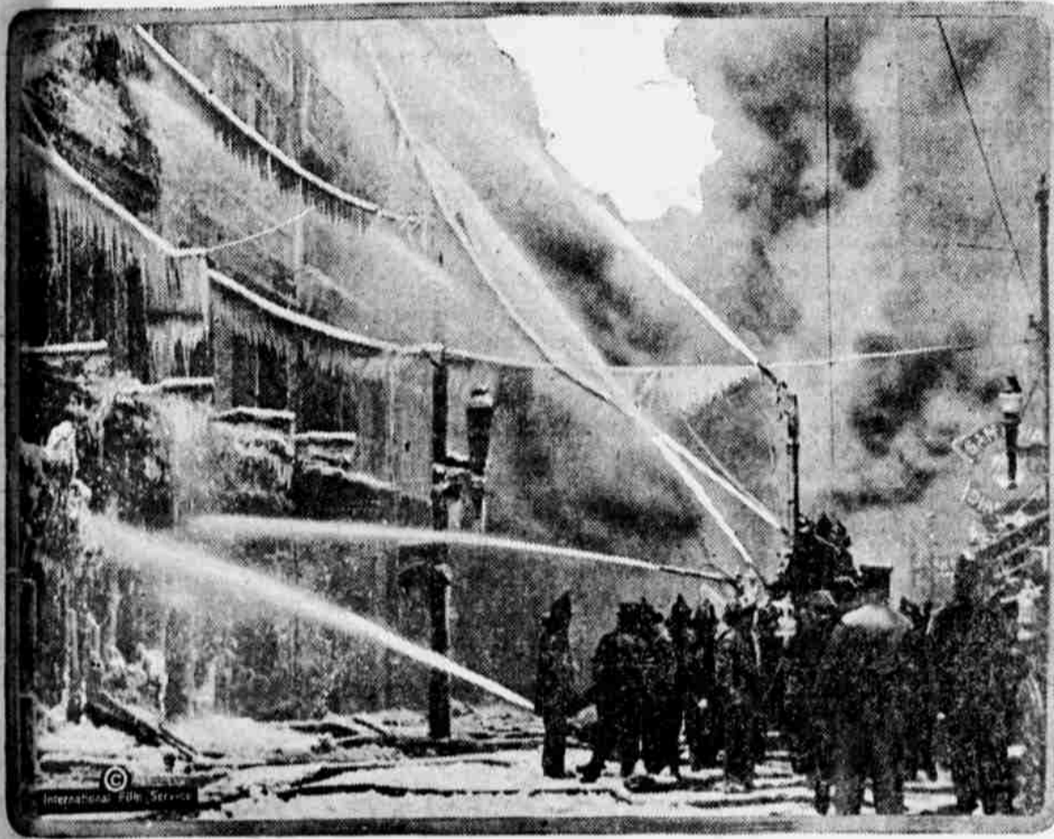
Scene during the recent conflagration in the business section of Pittsburgh, Pa., which resulted in the destruction of more than $2,000,000 worth of property.
