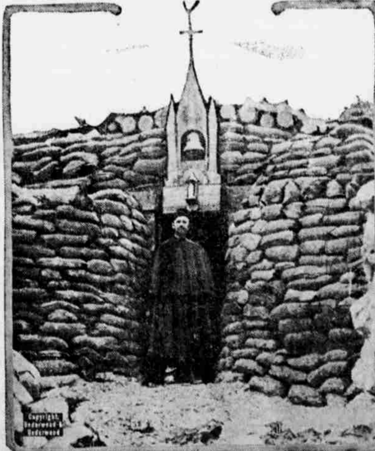
This French priest is rector of the quaintest sort of church on the Somme front. The church is built in a firing trench near Comblès and is protected from enemy attack by bags filled with earth. It is comparatively bombproof.
