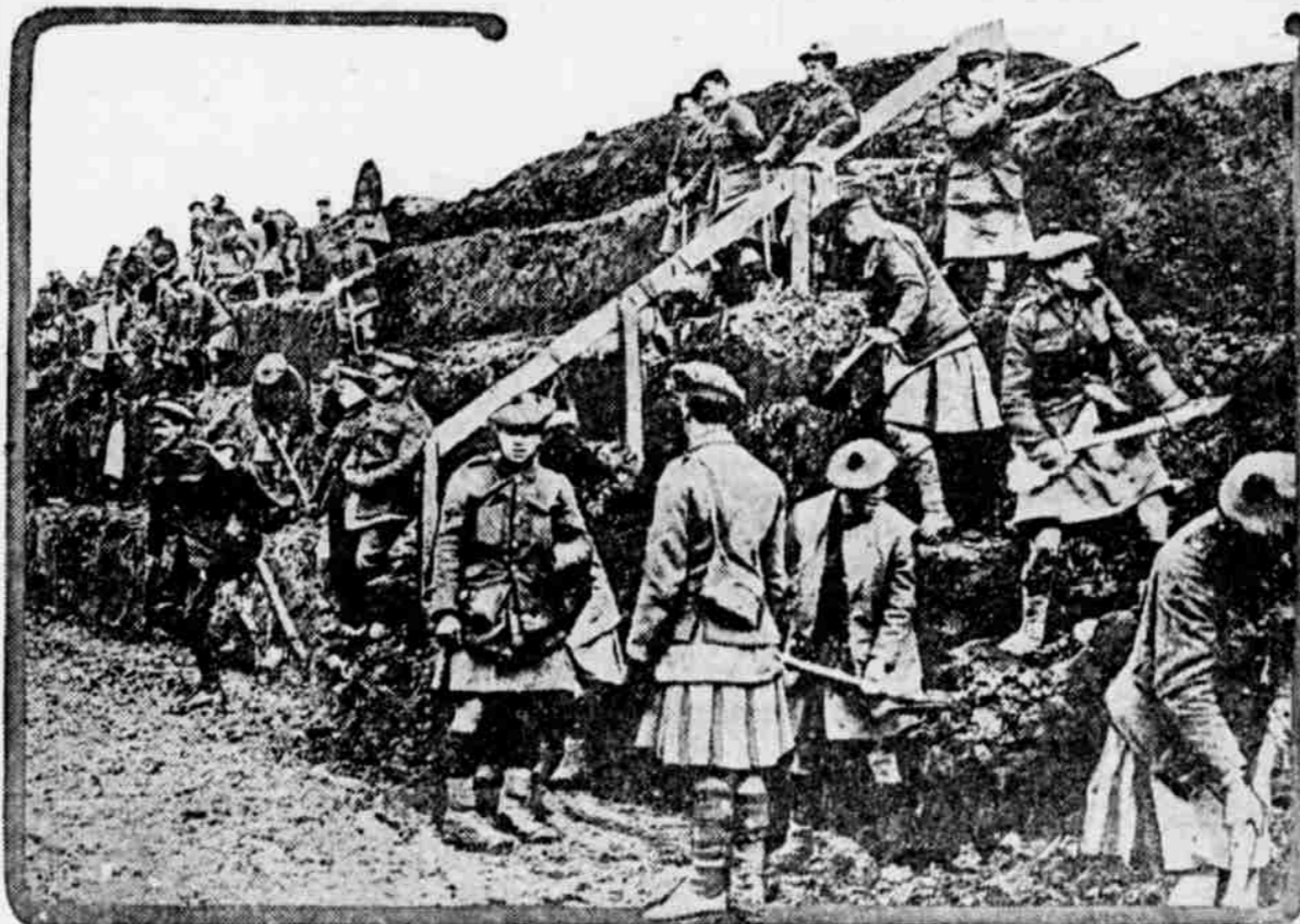
British official photograph taken on the western front, showing Scotch Highlanders at work in France broadening a military road. The Scots are eager to fight. Road-building is not to their liking, and they are only doing it as a warning-up to the deeds they expect to do later.
