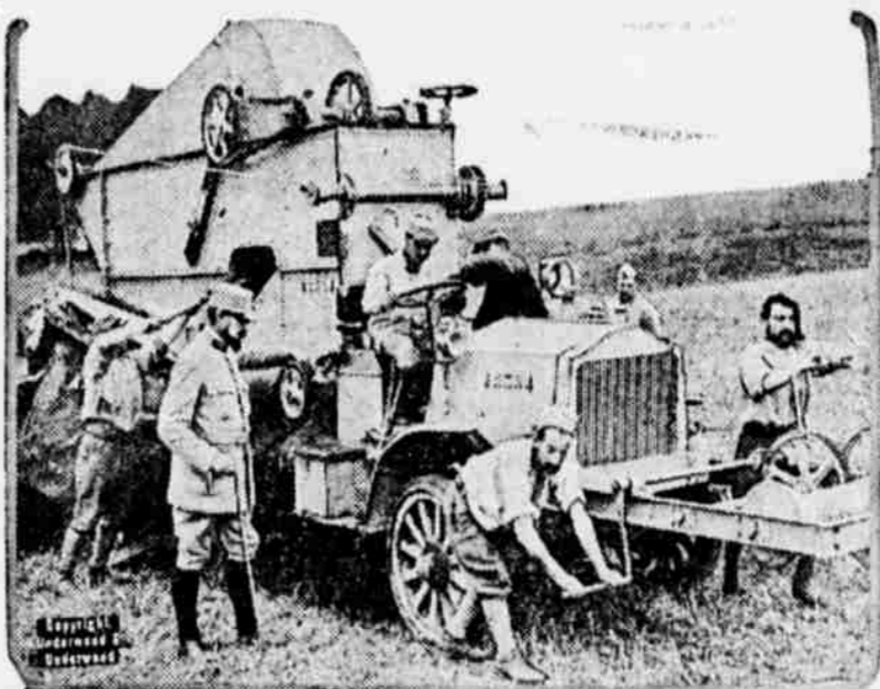
FRENCH MOTOR MACHINE DIGS TRENCHES
