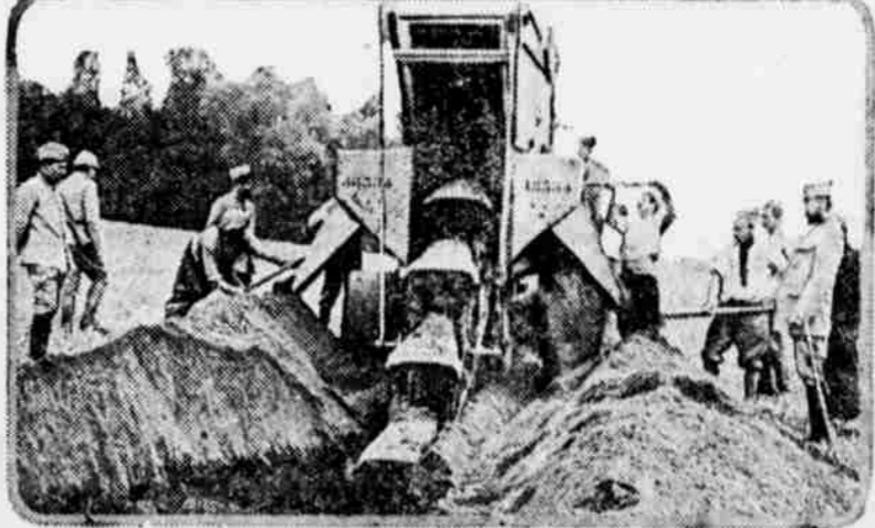
Upper: Side view of the powerful French tractor which builds trenches and constructs breastworks as it travels along. Lower: Rear view of the tractor, showing huge scoops which remove dirt, and other parts of the mechanism which does the work of scores of men.
