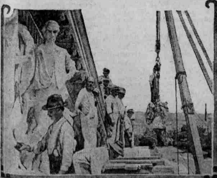
The laying of the final stone shown in the photograph completed the construction of the national capitol, which for more than 50 years has been unfinished. This was the last step in the construction of the pediment of the east wing of the house of representatives, a companion piece to the pediments over the main entrance and the senate wing. This portion of the house wing has been blank since the wing was nominally completed in 1857. An appropriation of $75,000 in 1908 provided for the final work of construction. This final pediment has been constructed by Paul Bartlett, who calls the design "The Democracy of the United States as Expressed by the Types of the Working People."
