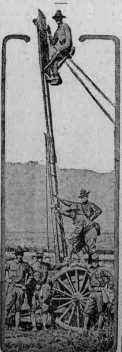
This photograph, taken in Mexico, shows one of the observation towers of the United States army in use.
