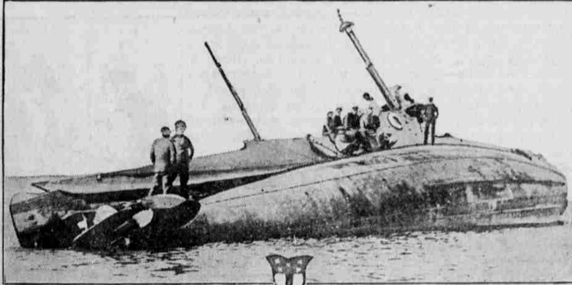
This photograph shows the submarine H-3 high and dry on a mud flat at San Diego, Cal. The H-3, one of the largest submarines in the United States navy, was just completing a half-submerged run in San Diego harbor when she struck the mud flat bow on at full speed and turned over on her port side. A mistake in location of the channel, which is deep enough to accommodate the largest sea-going vessel at low tide, is believed to have been the cause.
