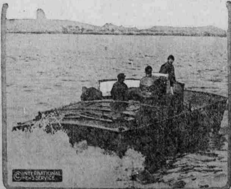
The "sea sled," which is said to have attained a speed of 75 miles an hour, photographed during its tests by the United States navy authorities. When running fast it coasts over the surface. It is intended to be armed with torpedoes.
