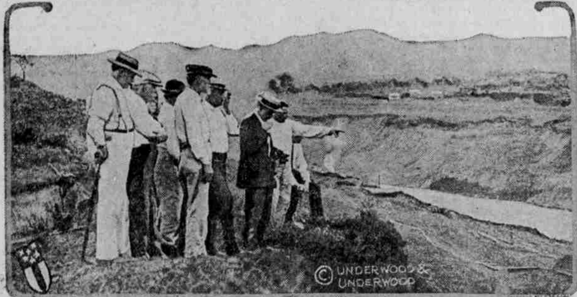
The great slides which have blocked the Panama canal have become a matter of such concern to the United States that President Wilson appointed a commission to study the causes of the slides. The photograph shows General Goethals and the commission viewing the slides and watching boats go through the canal.
