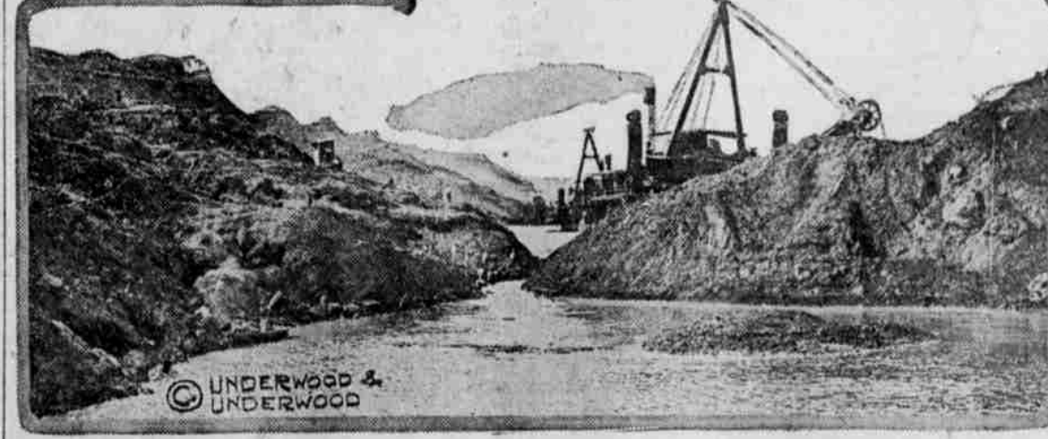
This photograph, taken October 26, near Gold Hill, pictures vividly the problem confronting the canal officials. Rock and earth have moved down from the heights on either side and forced the mud at the bottom up out of the water. In the foreground is an island which began to form just before the picture was made. It rose and spread until it joined the sides of the canal. The mass in the background, through which a narrow channel had just been blasted, came up first as an island and grew until it blocked the entire canal at this point. Shortly before this picture was made, a big blast had been shot off in the center and the water can be seen rushing through.
