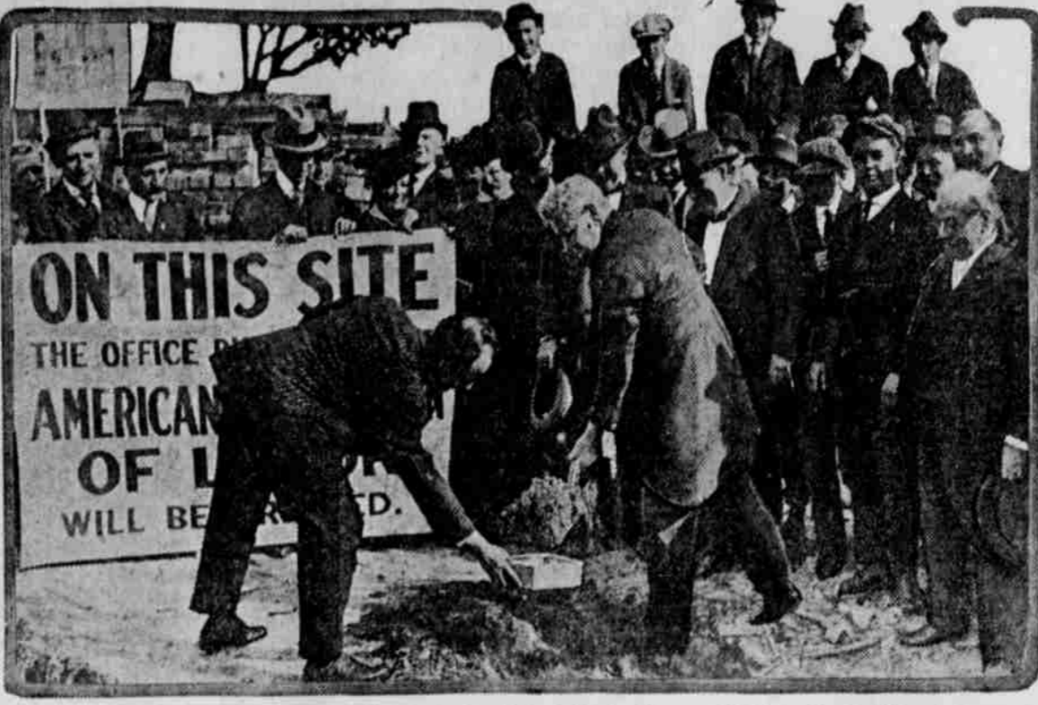
Secretary of Labor Wilson turning the first shovel of dirt for the new $200,000 office building to be erected in Washington for the American Federation of Labor.
