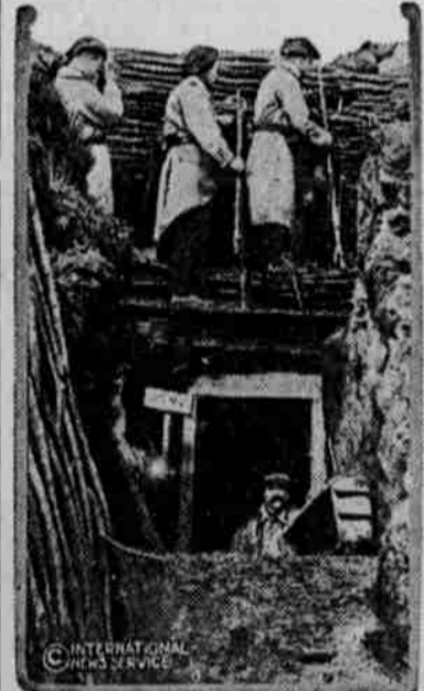
View of a French trench in the Argonne region. Above men are seen on the firing shelf, and below them is the entrance to one of the numerous saps.
