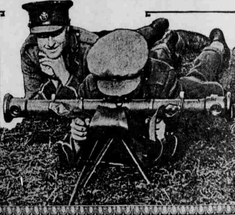
British observation officers with a range-finder noting the elevation at which the guns must be fired to strike the position of the Germans.
