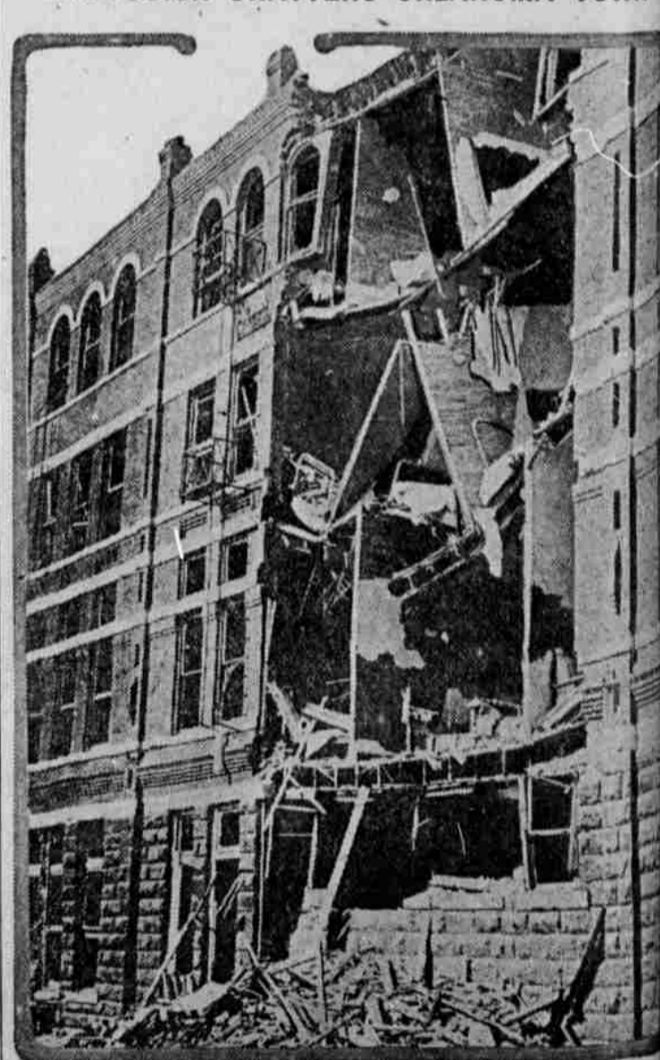
Many persons were killed or injured and great damage done to property in Ardmore, Okla., by the explosion of a tank car of gasoline and the resulting explosion of a quantity of dynamite in the railroad yards. This photograph of the east wall of the Whittington hotel shows how numerous buildings were shattered.
