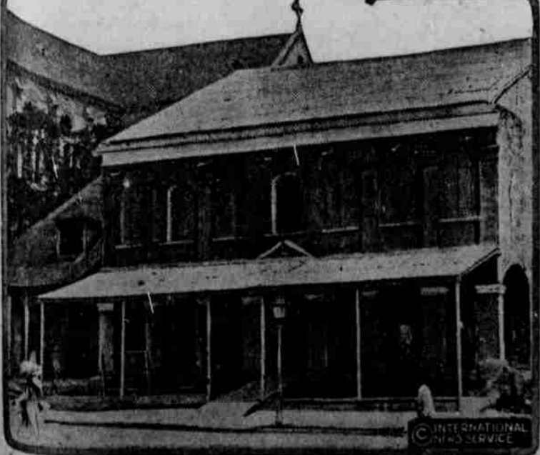
This is the antiquated jail at Port-au-Prince, Haiti, from which a large number of political prisoners were taken, lined up and shot by order of President Guillaume Sam, who was assassinated immediately afterward.
