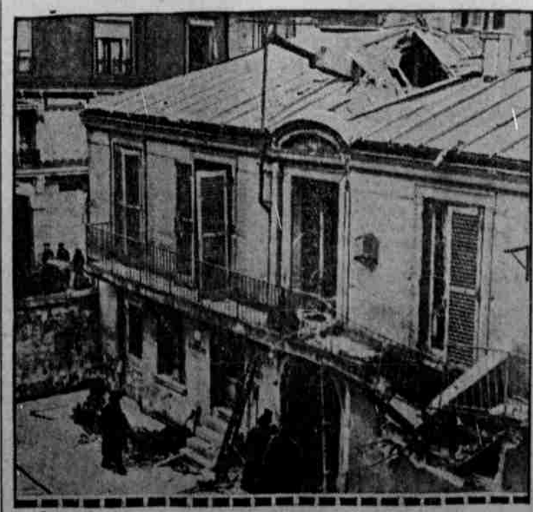
House in Paris partly wrecked by a bomb dropped from a Zeppelin during the recent airship raid on the French capital.
