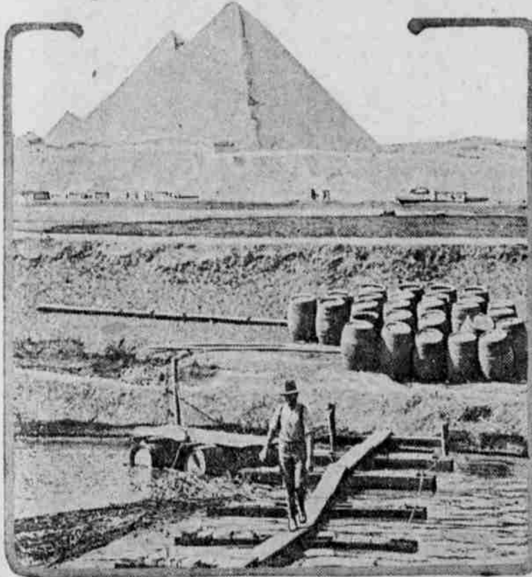
Plank bridge across an irrigation canal by the Australian troops near their camp by the pyramids of Egypt. The planks are supported by empty kerosene tins.
