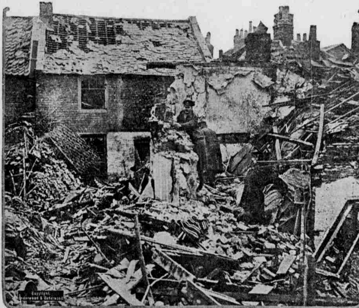
Houses in Albert road, King's Lynn, England, wrecked by bombs dropped from German aircraft that raided several coast cities on January 19.
